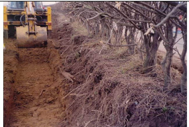
Trench excavated to rear of hedge.
