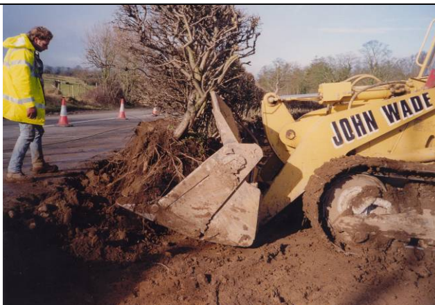
Sections lifted with 2m wide 4 in 1 bucket.
