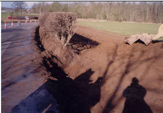
Trench excavated to roadside with back-hoe.
