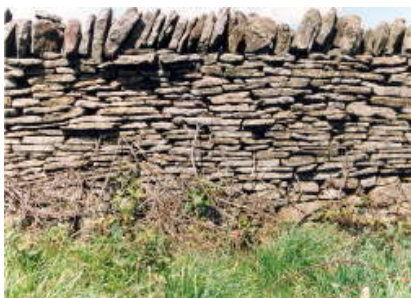
Wall of thin quarried stone
