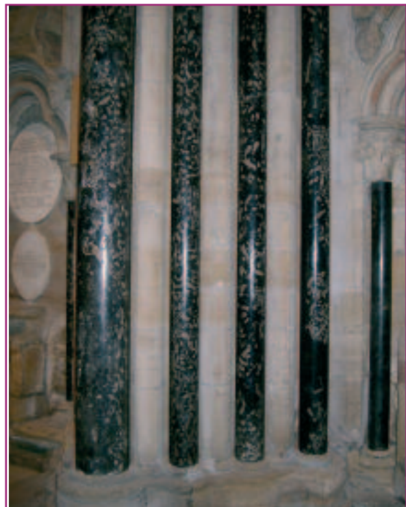
Photo 83. Durham Cathedral. Polished columns of Frosterley Marble contrasting with Coal Measures Sandstone in the Chapel of the Nine Altars.
