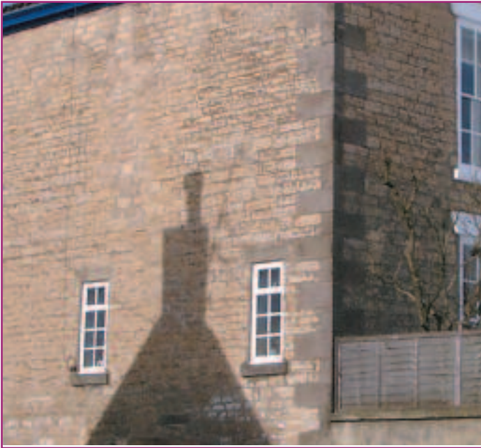
Photo 29. Heighington. Magnesian Limestone as a building stone: the quoins are Coal Measures sandstone.
