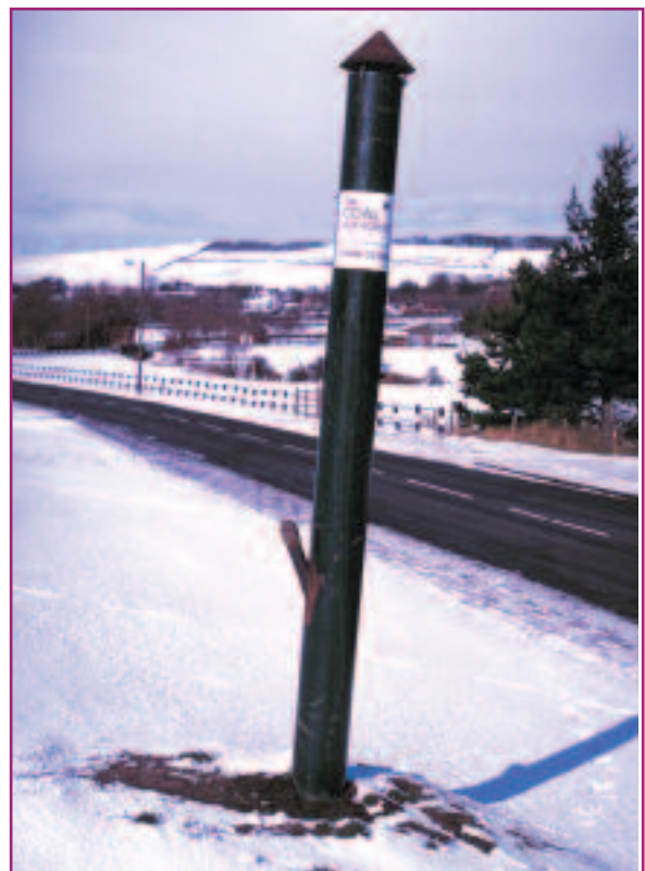
Photo 21. Gas vent to allow drainage of mine gases from old workings.
