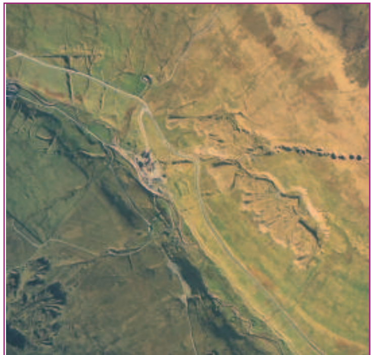
Photo 48. Aerial view of Groverake Mine, Rookhope. The course of Groverake vein is marked at the surface by a line of large crown holes.
