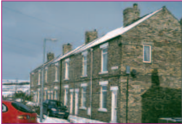
Photo 84. Helmington Row, near Crook. Pale grey bricks produced from Coal Measures fireclay.
