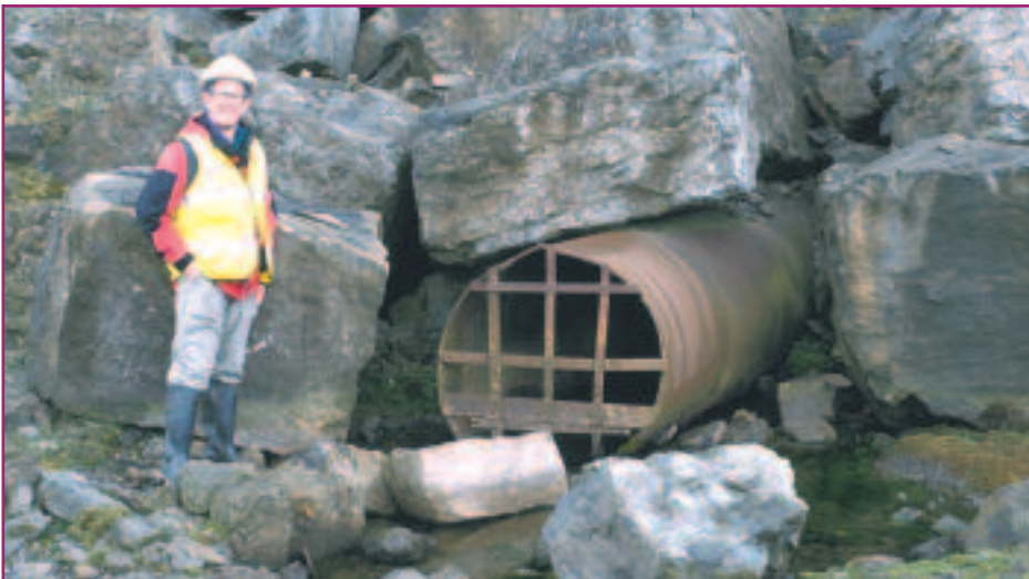
Photo 60. Entrance to Fairy Holes Cave in Great Limestone, Eastgate Quarry, Weardale.
